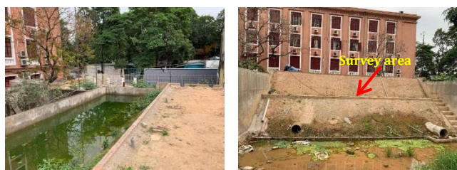
Figure 3: The artificial dam built at Thuyloi University for the SP measurement.
