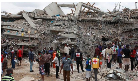
Figure 2: Middle view of the collapsed Reigners Bible Church
