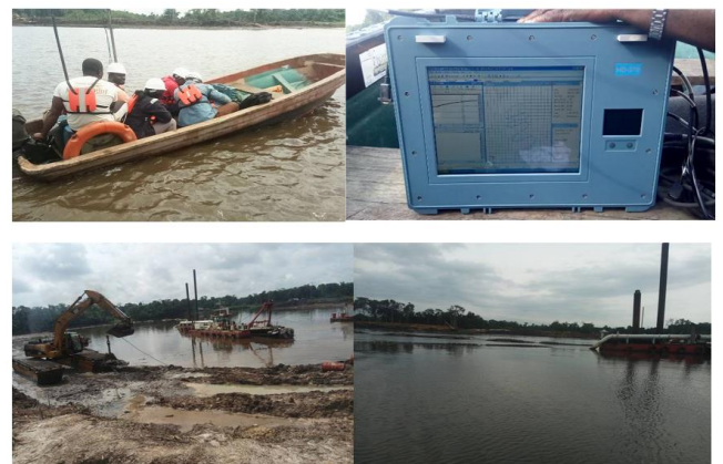
Figure 2: Bathymetric survey and dredging work in progress
